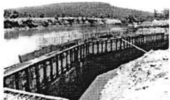
Work on the main canal
