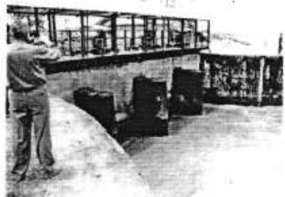
Head gate of main canal at Sejusa
