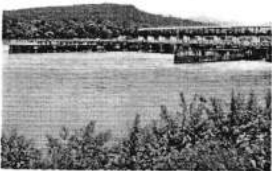
Barrage across Bordikorai river at Sejusa
