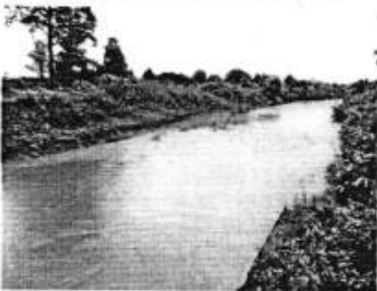
Main canal with water of Bordikorai river
